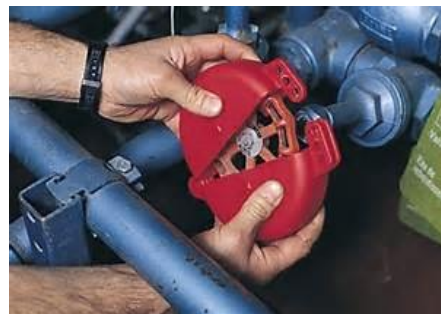
Figure 1 Valve isolator
