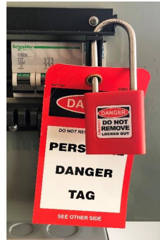
Figure 9 Circuit-breaker isolation
