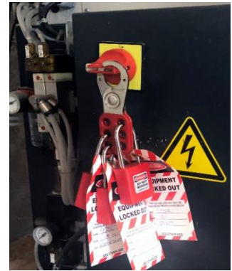
Figure 3 Use of scissor clasp for single point and several workers
